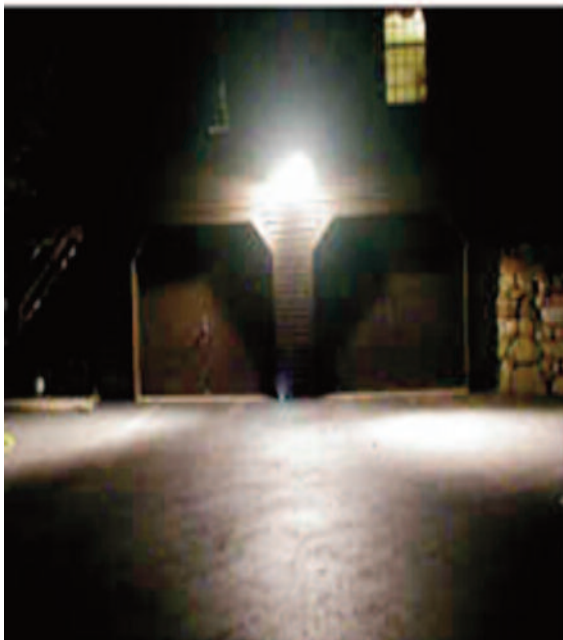
LIGHTS ON THE GARAGE TRAVELING UPWARD CAUSING SKY GLOW
