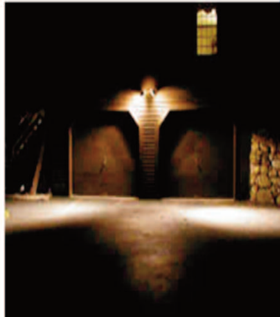
GARAGE LIGHT WITH A SIMPLE SHIELD TO REDUCE GLARE.
